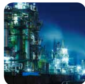
INDUSTRIALE INDUSTRIAL INDUSTRIEL
