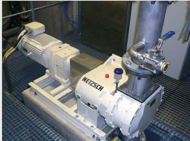
The TORNADO® T1 in use in a paper mill. Kaolin tankers are unloaded at 75 m<sup>3</sup>/h against a pressure of up to 4 bar.
