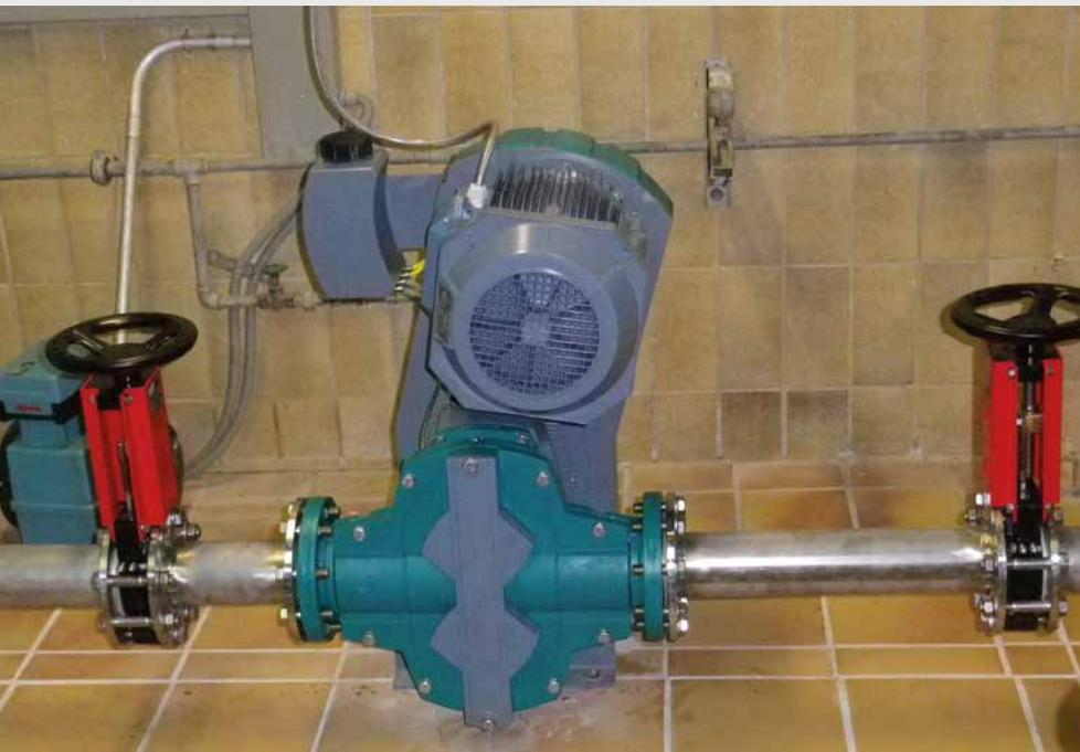
Used in a wastewater treatment plant, the TORNADO® T2 pumps sludge with 2% solid content at a capacity up to 18 m<sup>3</sup>/h against a pressure up to 2 bar.
