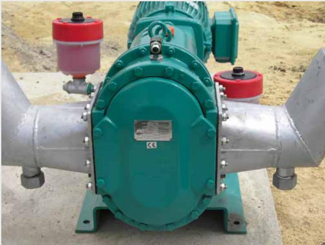
Feed pump for substrate in a biogas plant. Flowrate up to 40 m<sup>3</sup>/h at pressures up to 2 bar.
